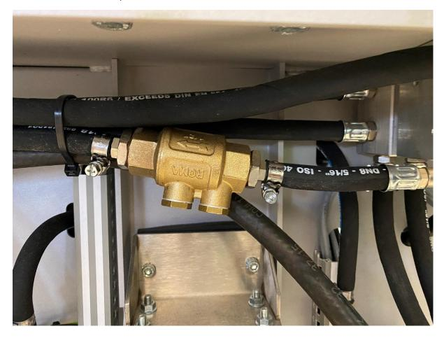
IMPORTNT check the arrow on the valve and connect to correct position
