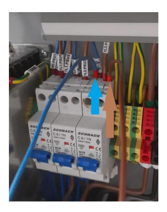
STEP.6 (Remove the sticker on the new part and insert as shown in the picture)
